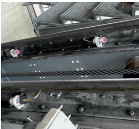
Several lubricators are installed on a cable saddle. Installation is simple thanks to the use of a magnetic clamp.
