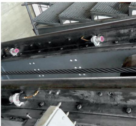
Several lubricators are installed on a cable saddle. Installation is simple thanks to the use of a magnetic clamp.
